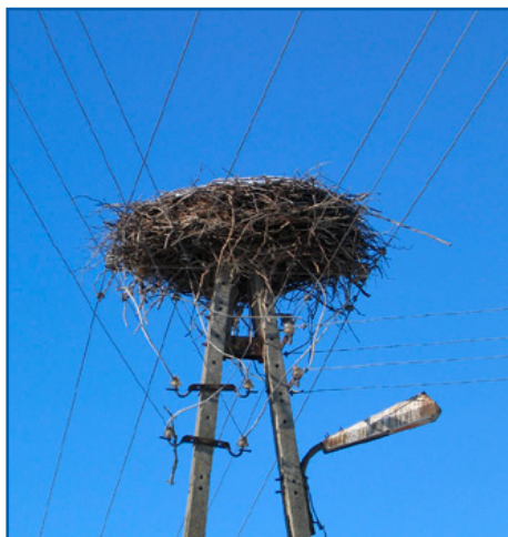
Nest on a power line with “bare” wires. Photo: AT
