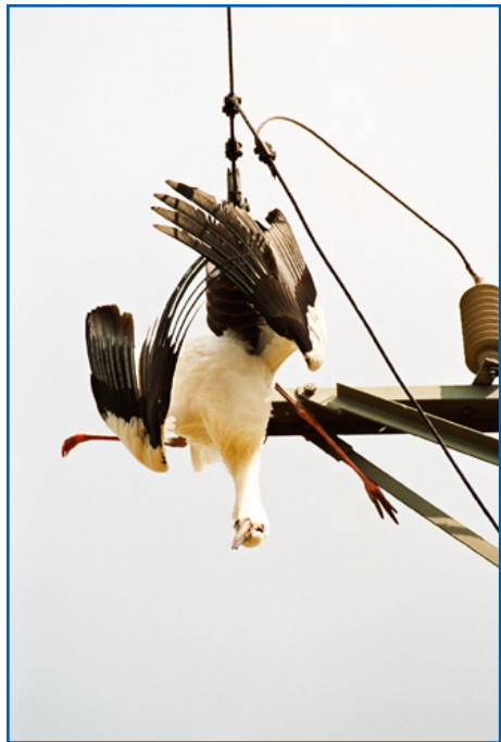
An inadequately secured pole can be the cause of death of many storks. Photo: MR
